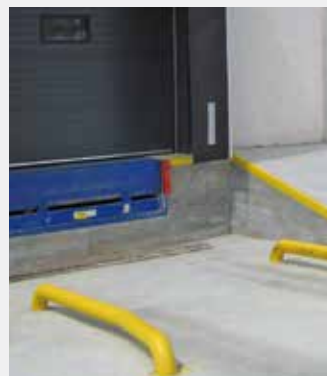
G-25 in steel painted yellow set in cement.
