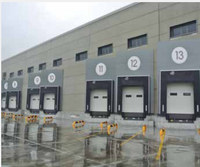
HIDRA leveler with dock shelter AB and truck guides G25 .
