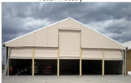
Instant Pass in hangar for aircraft - with removable legs – total opening 40 m
