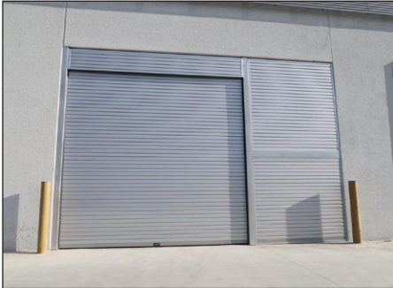
ROLLER SHUTTER DOORS
