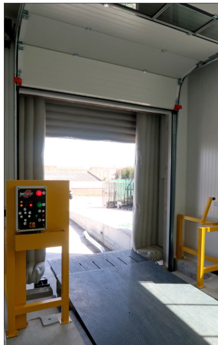
Outside and inside view of Isoperfect loading dock with inflatable shelter colour grey
